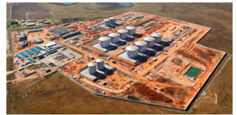
New Multi-Purpose Pipeline (TM1 & TM2)
